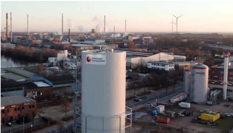
Hamburger Energiewerke warm water buffer tank
