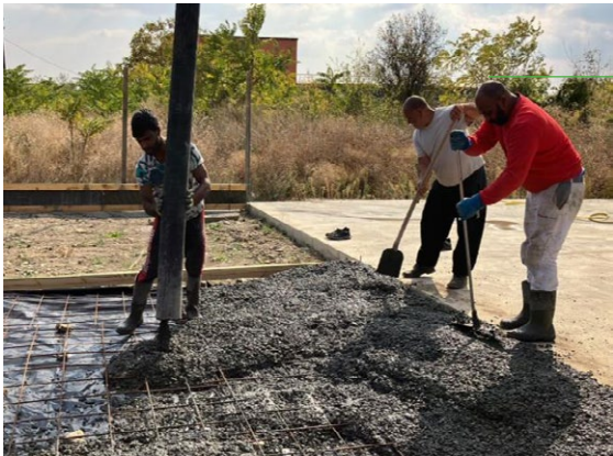
Floor slab of a private house
