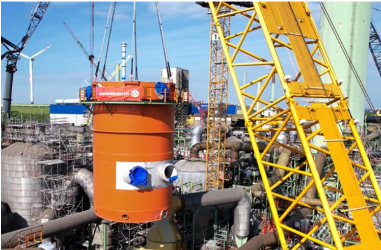
Retrofitting the contact acid plant in the Industrial Heat project
