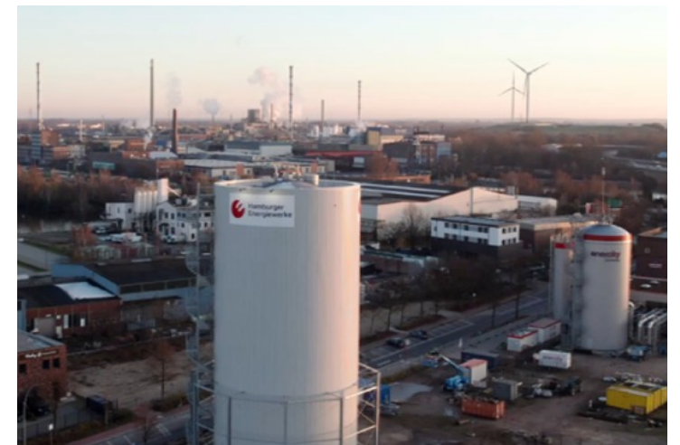
Hamburger Energiewerke warm water buffer tank
