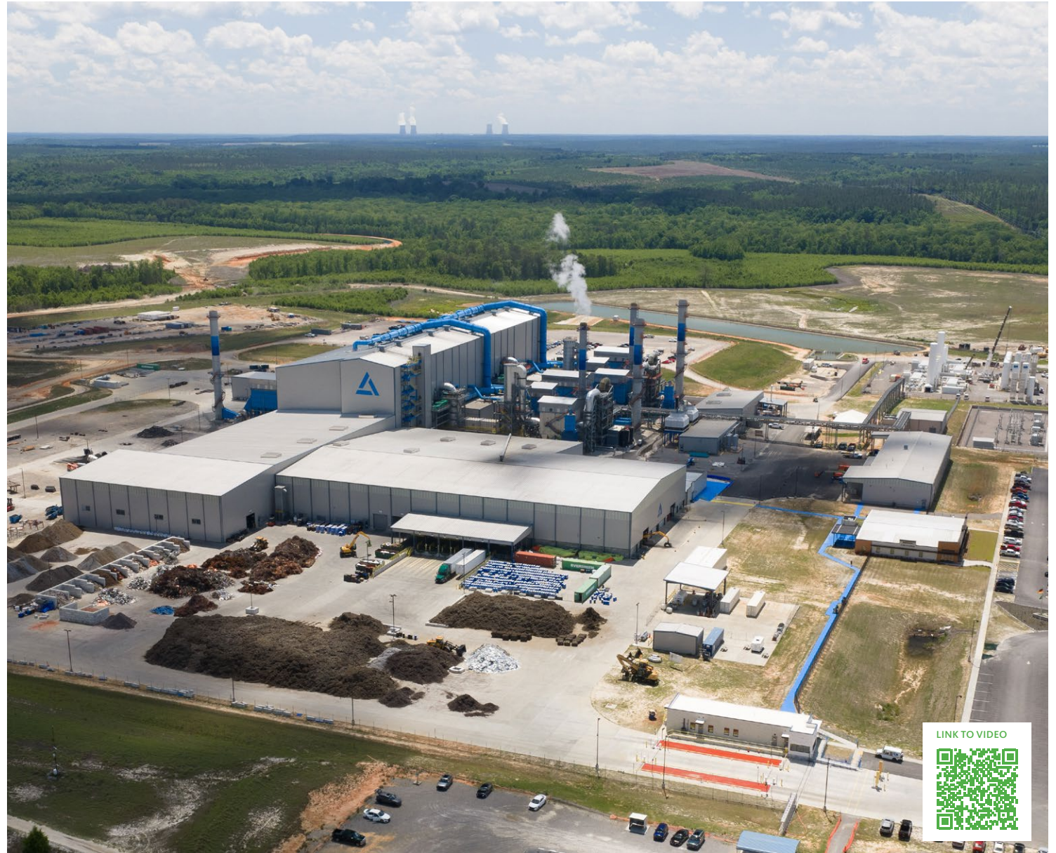
The site at the beginning of December 2024
