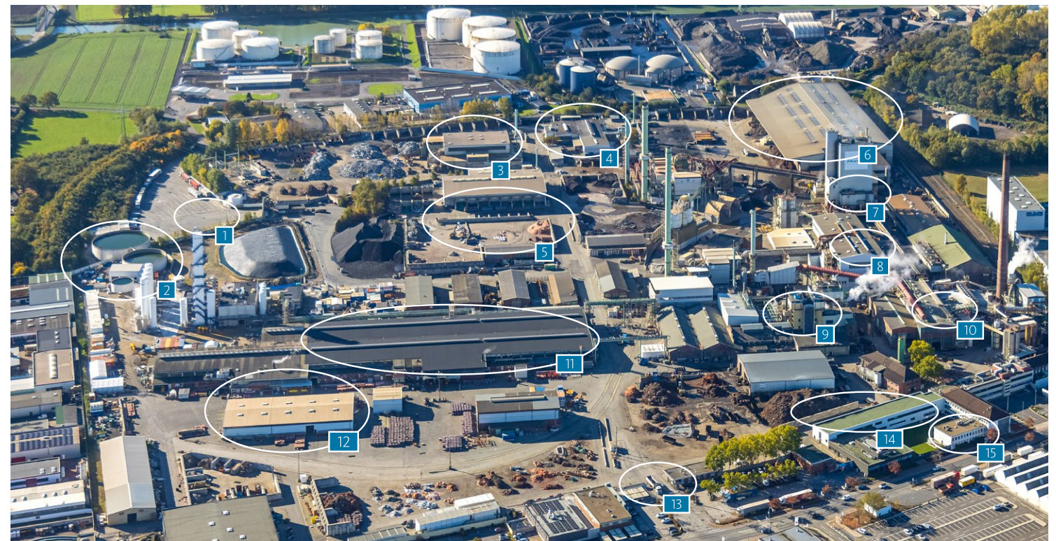
Fig. 3.1: Overview of Lünen site facilities
