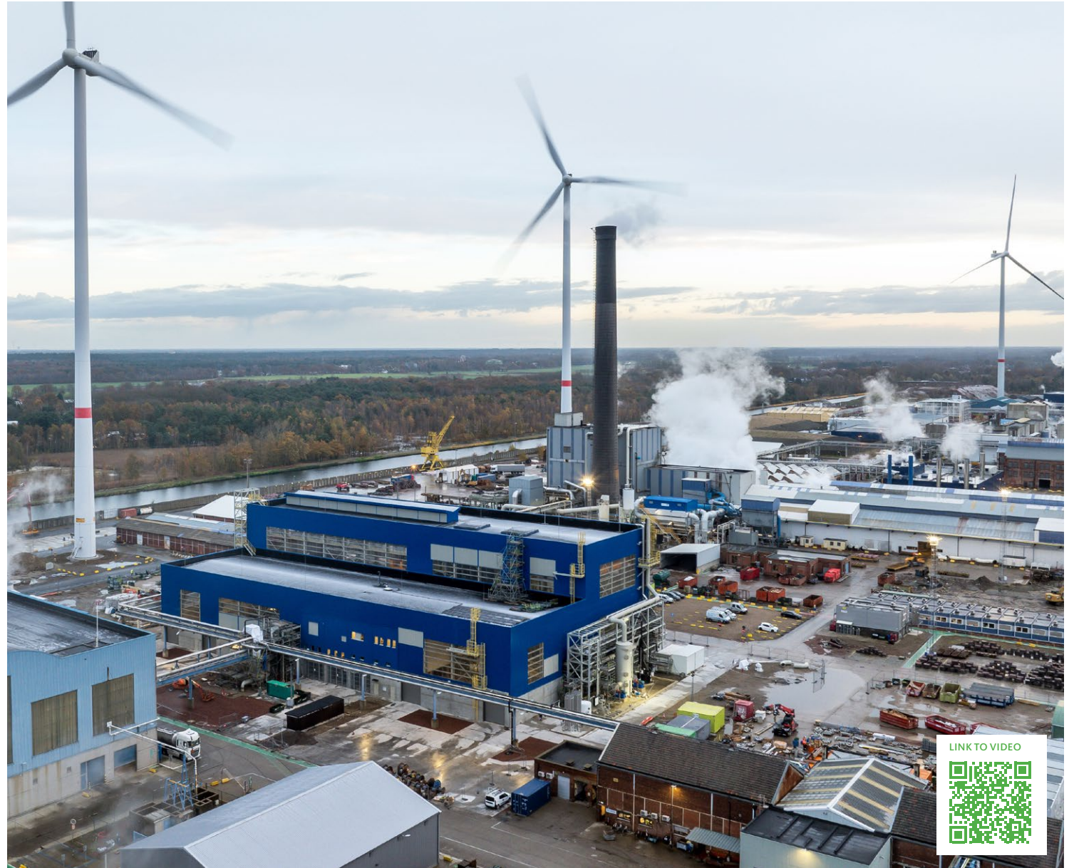
The new facility under construction in early November 2024
