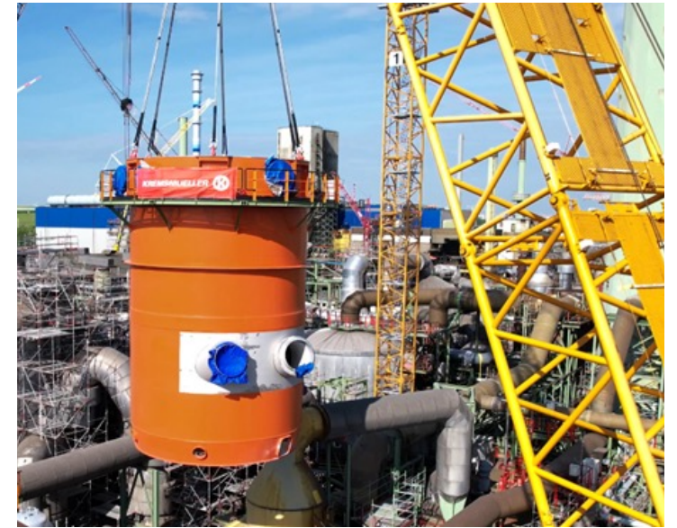
Retrofitting the contact acid plant in the Industrial Heat project
